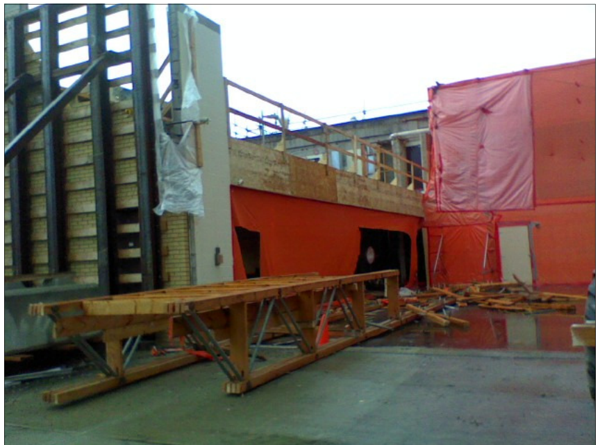
Trusses removed from Mezzanine
