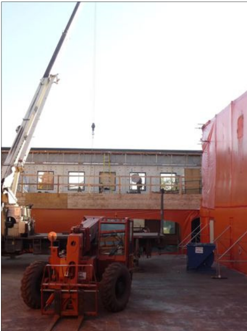
Crane at work
